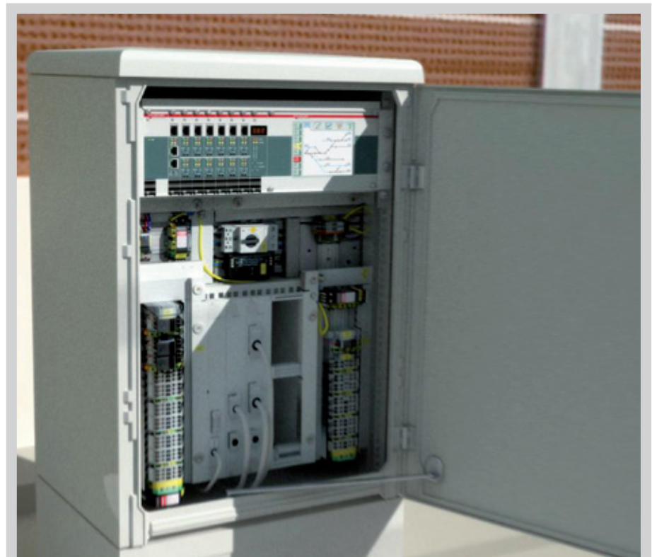
Figure 7: The components of the FAdC are suitable for use in compact outdoor cabinets along the track.
